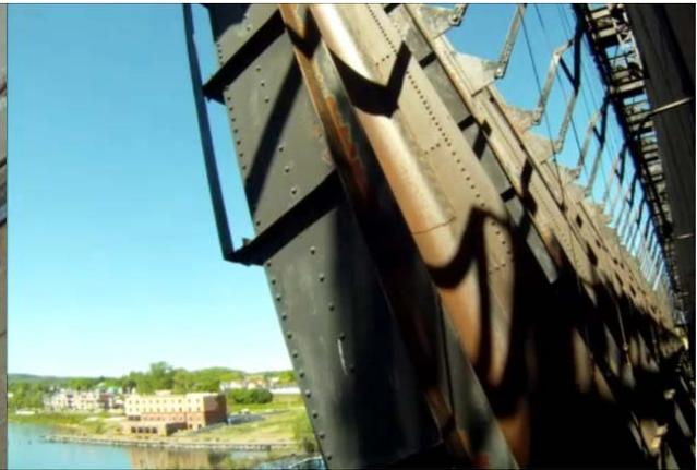
*Photo 4-14: Typical view of chute on south side showing riveted steel construction.*
