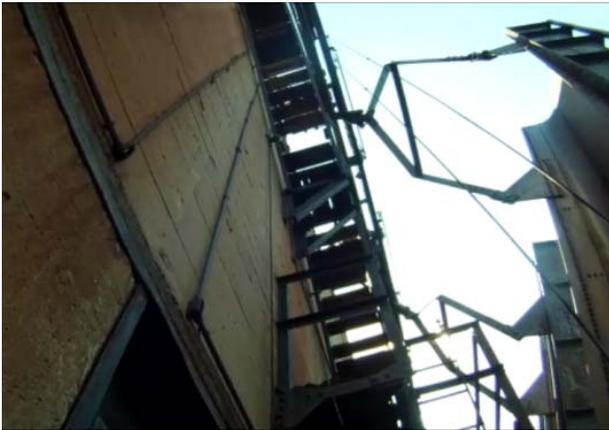
*Photo 3-21: Looking up at bottom of stairs on north side. Note good condition of pocket wall.*
