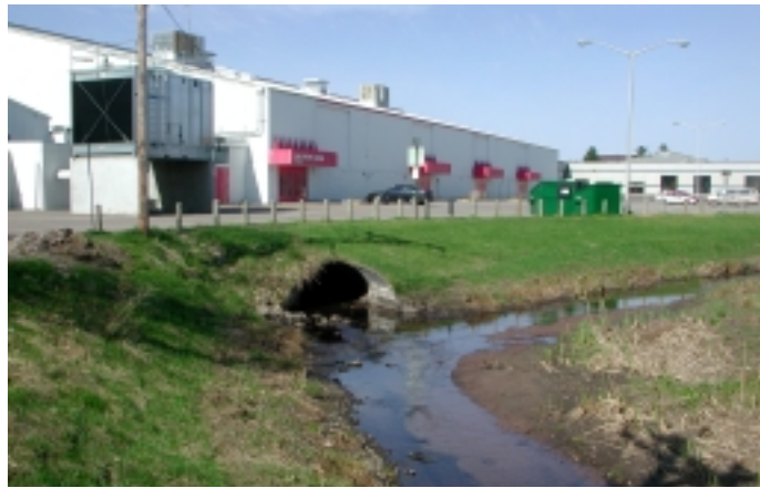
Storm Drain North of the Marquette WTP
