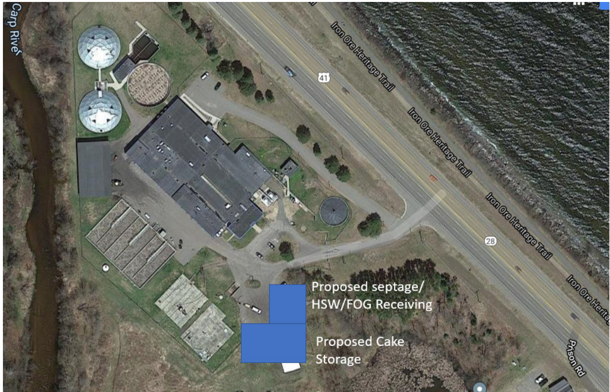
Figure 1: Aerial Photograph of the Marquette WWTP showing the location of the proposed improvements.
