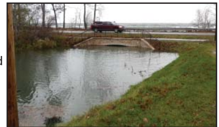
Pictured above: Lakeview storm drain project site
