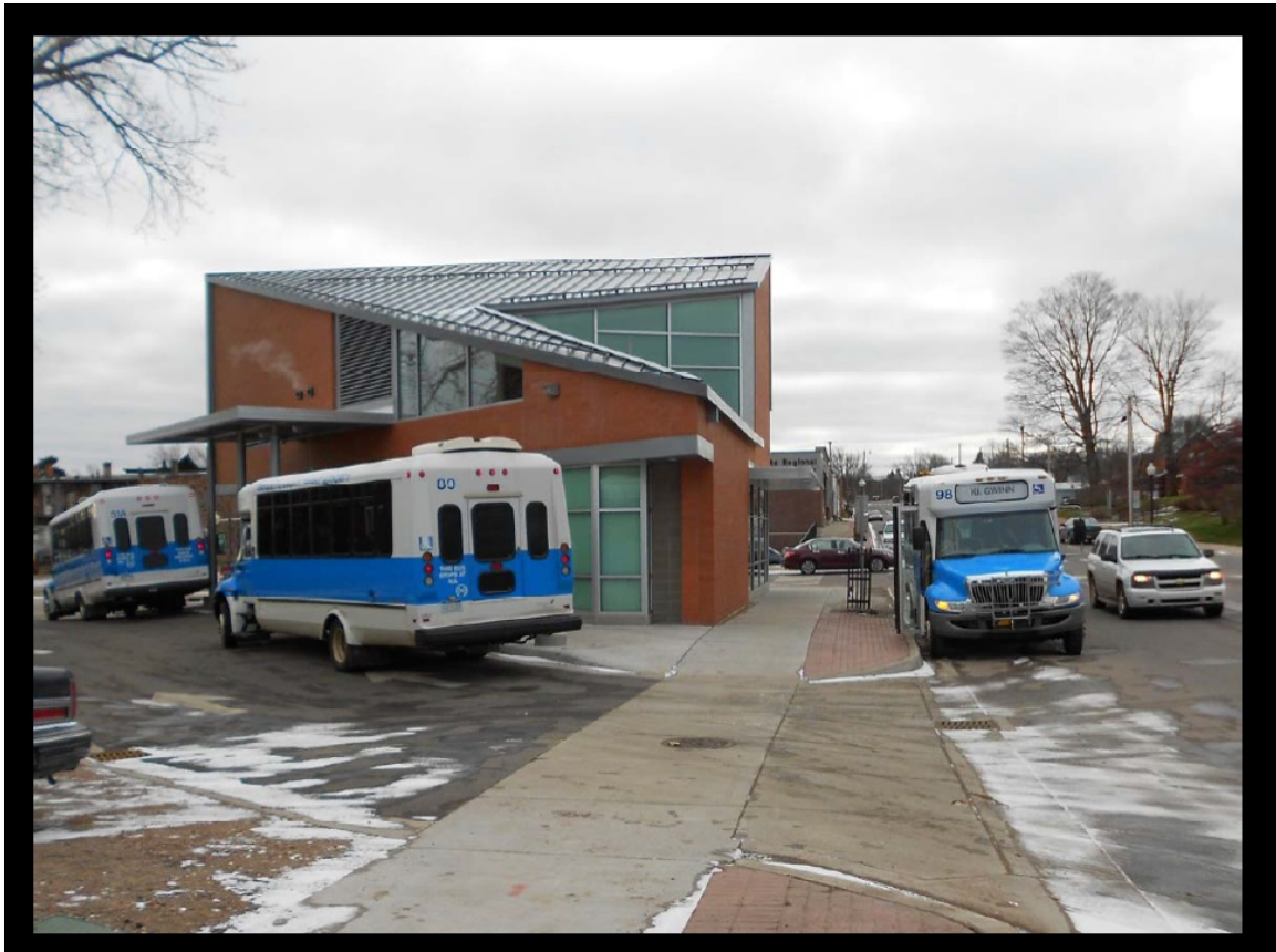
Figure A-4: New Marq-Tran Downtown transfer station at South 3 rd and Spring Street
