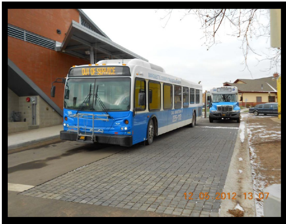
Figure 3-2: Marq-Tran busses at new Downtown transfer station
