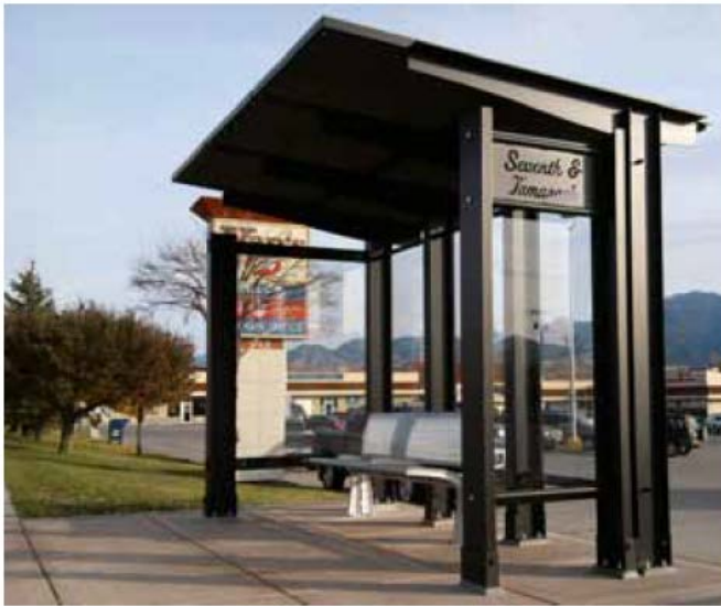
Figure 21: Locally designed and sourced bus shelter in Bozeman, Montana. Cost estimate: $17,000 including installation, concrete pad, trash receptacle, and bike rack.
